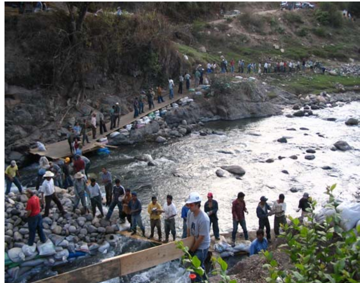
Construction of the Motagua Bridge in Guatemala (Recent EWB Project)
