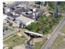
47th Avenue Bridge
